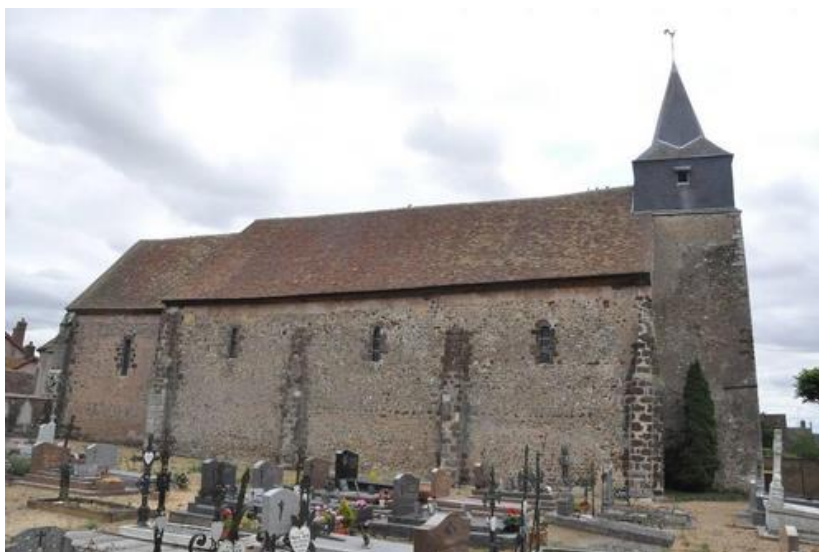
Figure 2 Saint-Gilles de Charonville, murs nord
